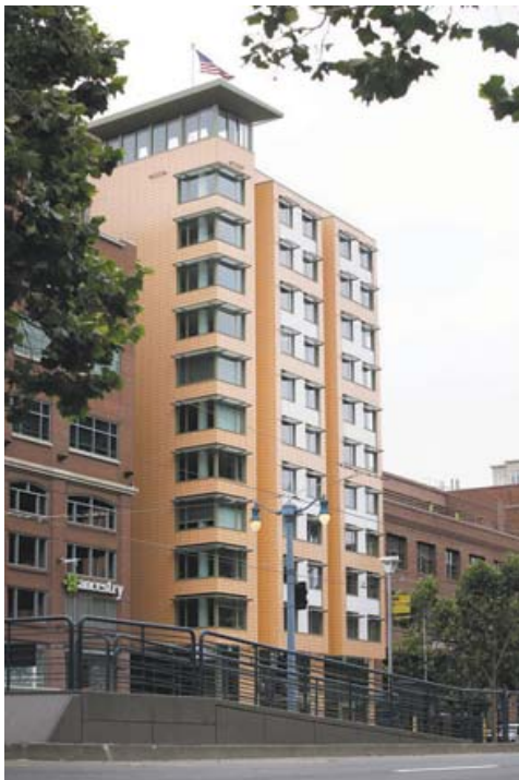
The 159-room hotel is clad mainly in tiles of earthy terra-cotta and topped by a narrow crown.
